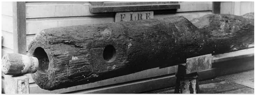
Excavated old wooden water pipe. Note the original fire plug to the left.
