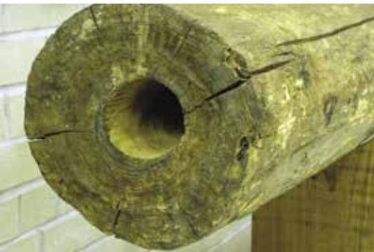
Early Wood Water Pipe. Photo courtesy Firefighters Association State of New York Museum of Firefighting.
